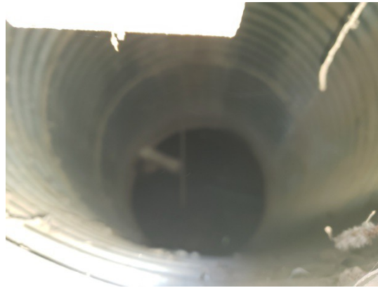
Exterior uncovered lip of drain and cover. Interior photo taken with camera probe. Found to be Dry.
