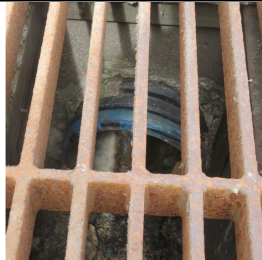
Storm Drain grate SW corner 23.5 feet.
